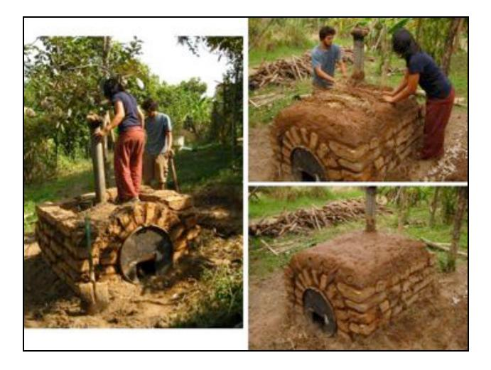
The kiln was loaded with wood packed as tightly as possible. A log laid across the bottom supports the wood and provides space for airflow from the inlet into the center of the kiln.
