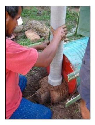
Use a generous amount of sticky cob to seal the chimney pipe to the bottom of the drum.
