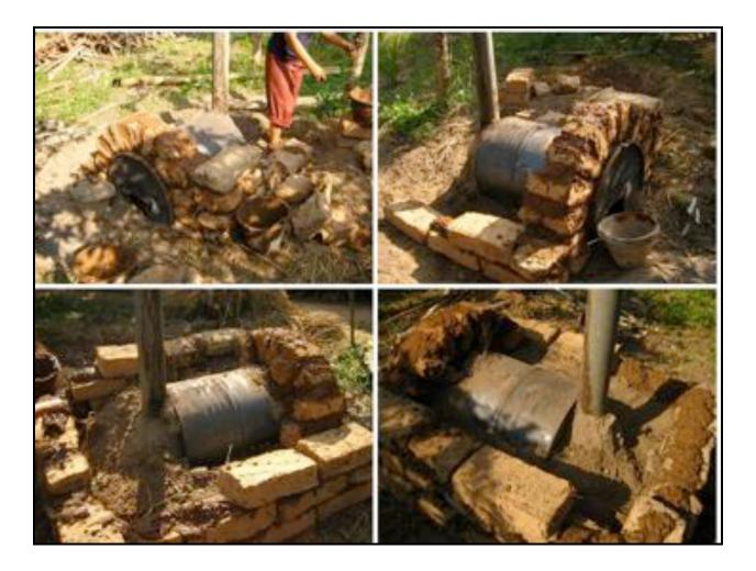
The earth was well tamped and covered with a thick layer of straw for insulation. A cob plaster was applied to cover the straw.
