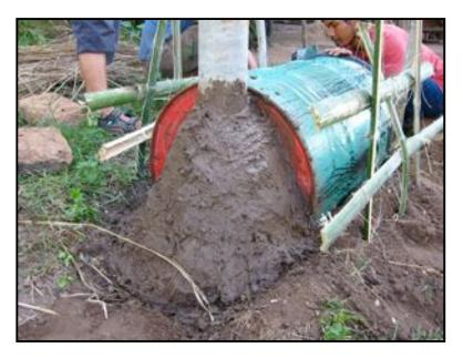
The easiest way to insulate the kiln is to make a simple bamboo structure around it and backfill with earth, sand and straw.
