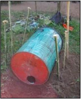
Using some adobe bricks and cob (a mixture of mud and straw), connect the chimney pipe to the outlet opening in the bottom of the drum.
