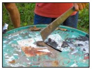
Cut a round hole in the bottom of the drum approximately 15 cm in diameter. Lay the drum on its side in a shallow excavation.
