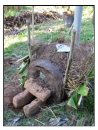
An inlet is made with adobe bricks, and the lid plastered with mud for insulation and to seal the kiln.
